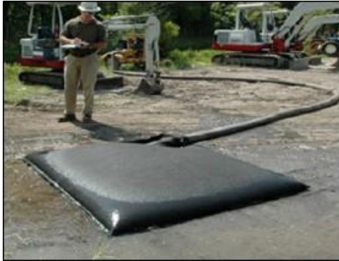
Plate 2-1 Silt Bag with water being pumped through
