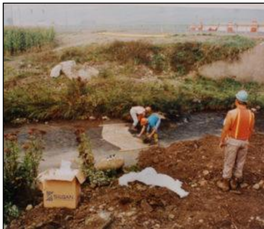
Plate 2-3 Typical Sedimat Details (Source: https://www.hy-tex.co.uk/ )
