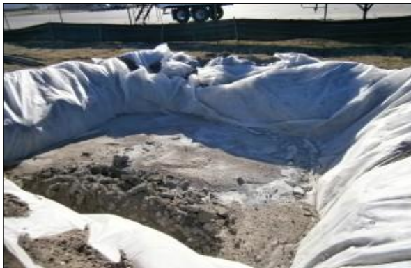
Plate 3-2 Concrete washout area
